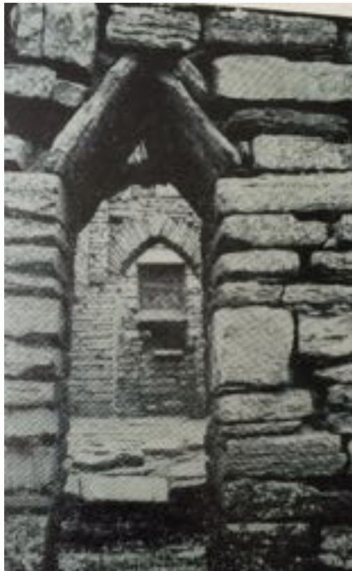
Figure 18: Triangular arch of the western porch doorway of the Eynhallow church. The form is found in Anglo-Saxon architecture, including St. Peter's church in Barton-upon-Humber. From: Mooney, Eynhallow , 155.
