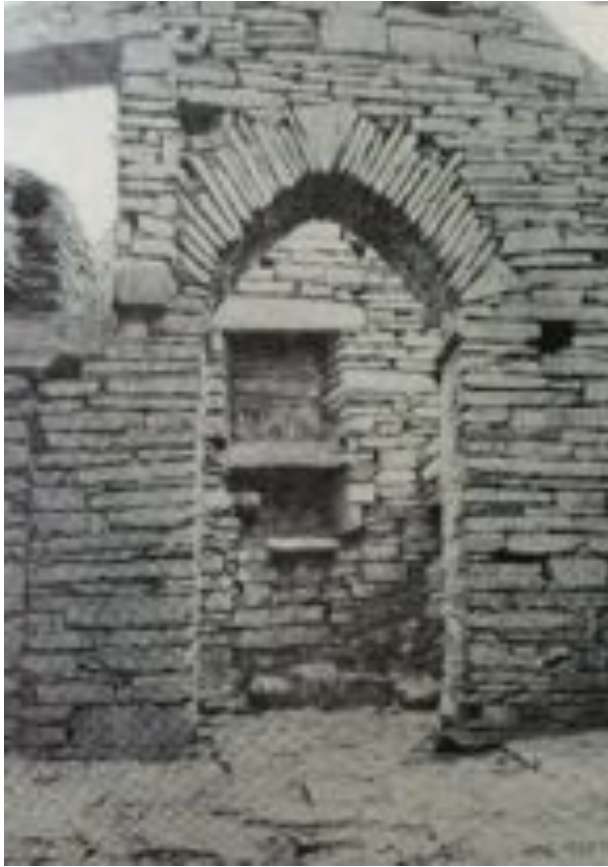
Figure 19: Pointed arch into the chancel of the Eynhallow church. While the pointed shape recalls the architectural trends in Britain and Europe starting in the twelfth century, the construction method is unique. With three triangles acting as the two springers and keystone, the rest of the arch is filled in with undressed freestones that would have necessitated some type of centering or support. The only other arch that uses three triangles in this way is found in Hvalsey, Greenland. From: Mooney, Eynhallow , 159.
