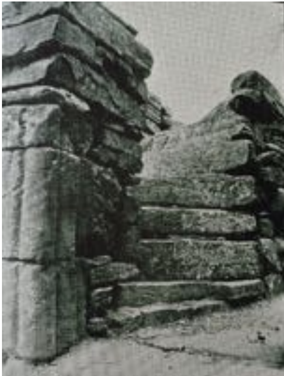
Figure 20: Entryway and steps to the Eynhallow belfry. The stones of the lower doorway have been dressed to resemble columns. From: Mooney, Eynhallow , 153.
