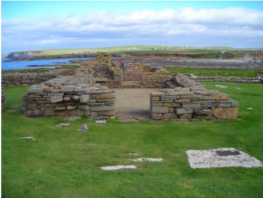
Figure 15: Church ruins on the Brough of Birsay from the West. Projecting stones around the doorway suggest a tower was planned, but never completed. Author's photograph.
